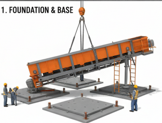
Modular Base Frame Installation
