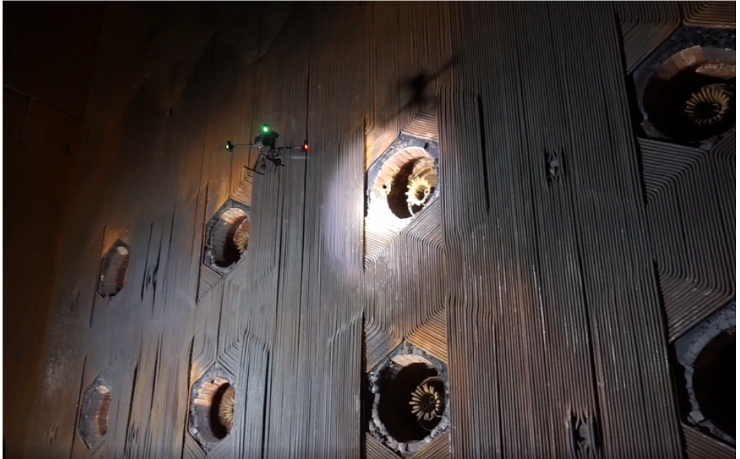
Figure 1: Autonomous inspection of the furnace of a thermal power plant using the developed navigation module and DJI Matrice 300
