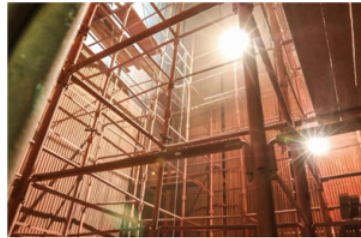
Figure 3: Scaffolding in the furnace boiler of thermal power plants
