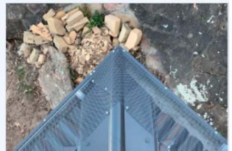
Chimneys Activate Window Go to Settings to activate
