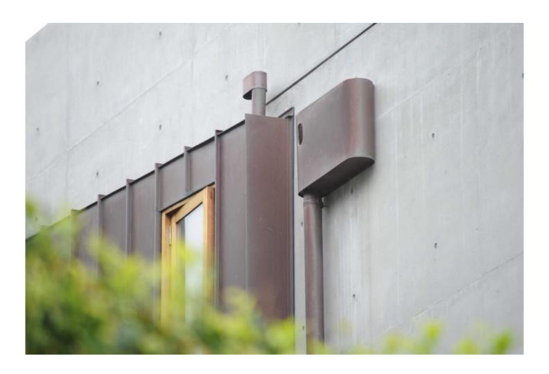
**Pune, Jun 25, 2019 (<u>Issuewire.com</u>)** - **Rainwater** heads are used to keep water away from the roof and fight against potential water damage stemming from rainfall.
